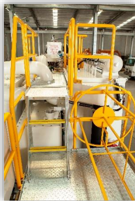
Image 35 - Walkway and Handrails on top of the debris tank
