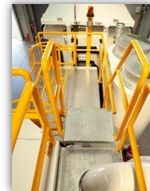
Image 38 - All handrails painted safety yellow
