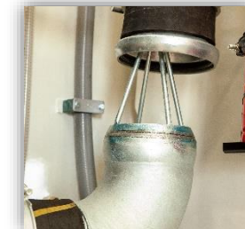
Image 5 - Proprietary manifold to allow maximum airflow whilst minimising intake noise and vibration
