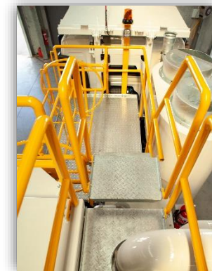
Image 38 - All handrails painted safety yellow and to Australian specification
